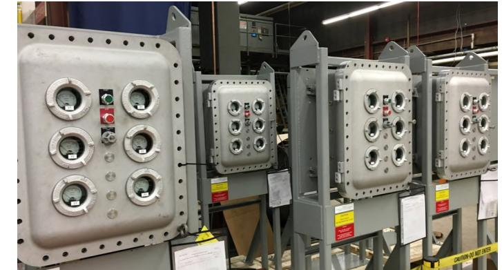
Level Switch - one per desalter. Safety interlock, wired normally open allows the power units to energize only when the technology host vessel is liquid full
